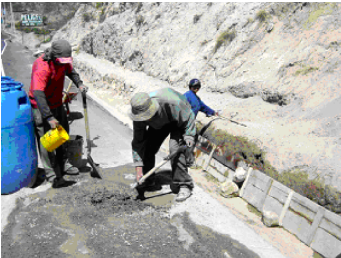
Repairing a ditch in Ecuador
